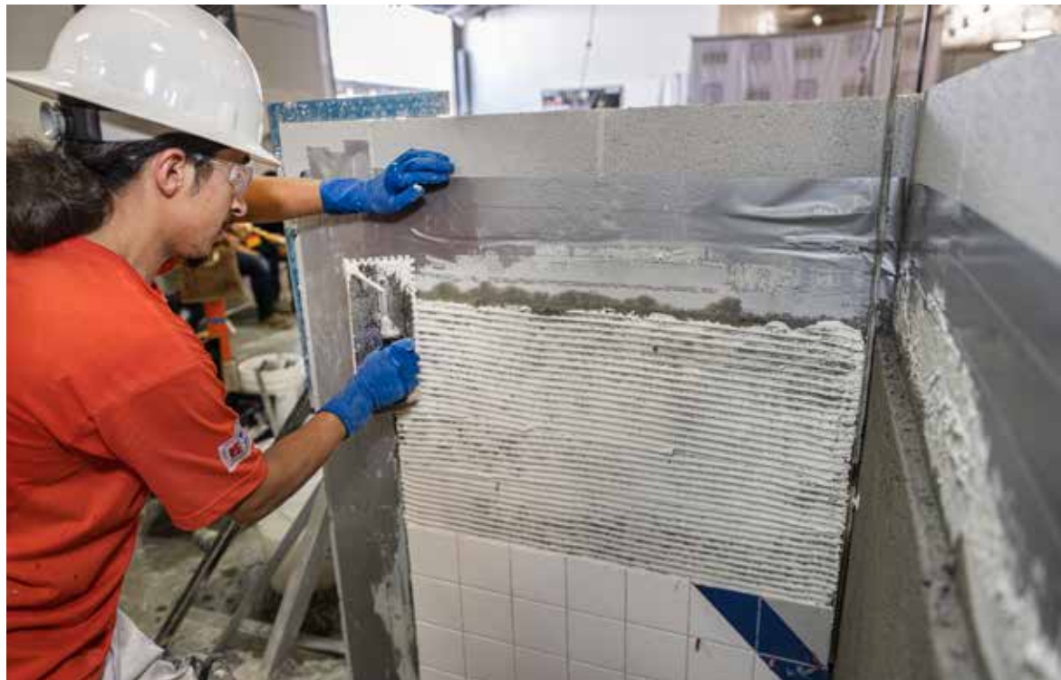
Vito Torres applies thin-set mortar with a quarter-inch notched trowel.
