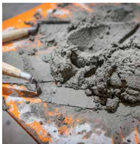
Brick mortar is mixed and ready.
