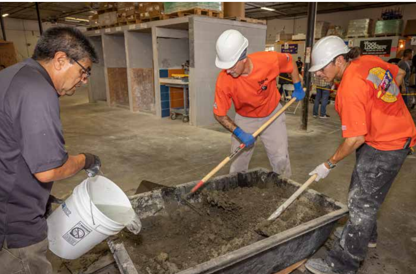
Tile instructor Luis Torres, left, helps mix up dry pack for a tile base.
