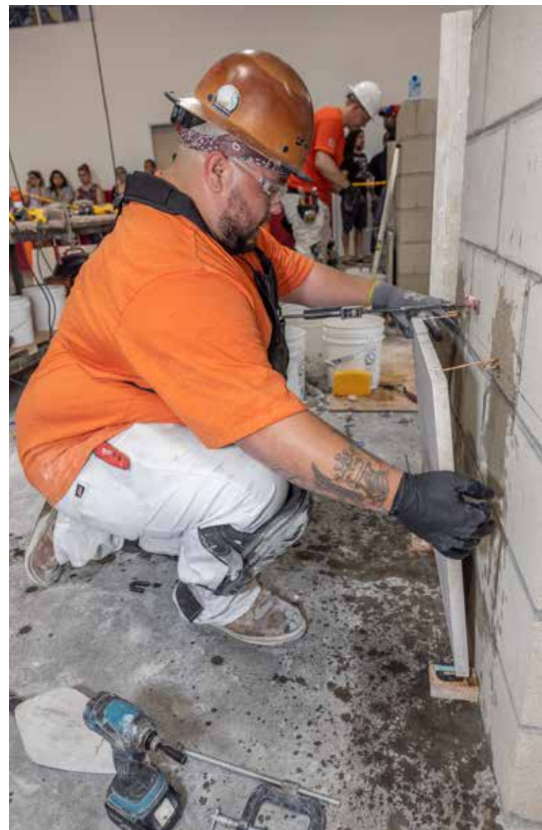
Torres will complete his task by filling the holes with casting plaster.
