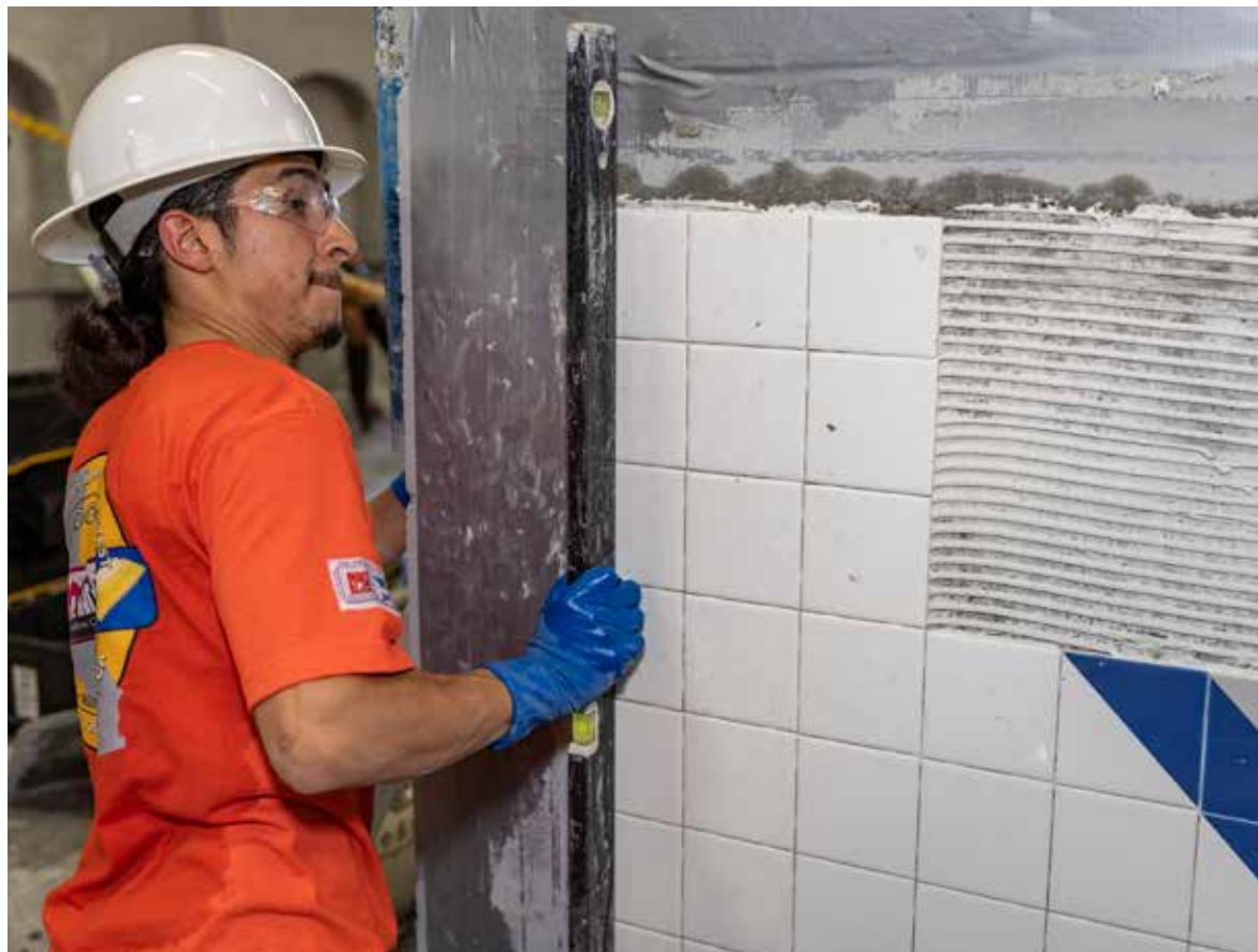
Torres uses a level to check his work.
