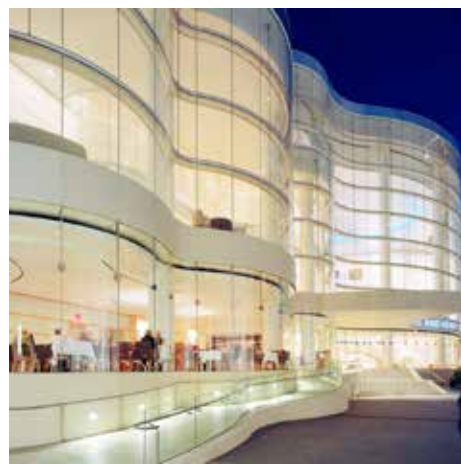
Segerstrom Concert Hall, a Costa Mesa attraction, won the Q Award for union construction.
